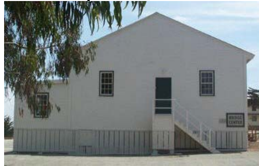
Building 2925: After Encapsulation
