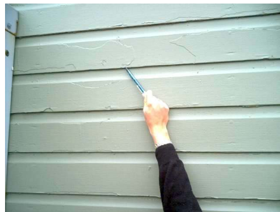
Detail of West Wall
