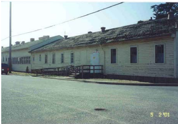
Building 2286: Before Encapsulation
