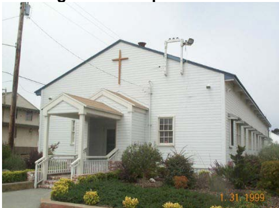
Building 2233: Scraped and Painted
