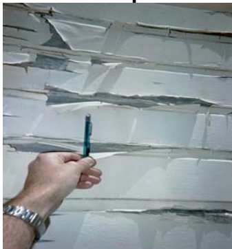
Large Paint Chips Before Encapsulation
