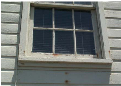
Large Paint Chips Before Encapsulation
