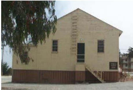
Building 2925: Before Encapsulation
