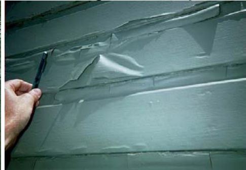
Detail: Large Paint Chips
